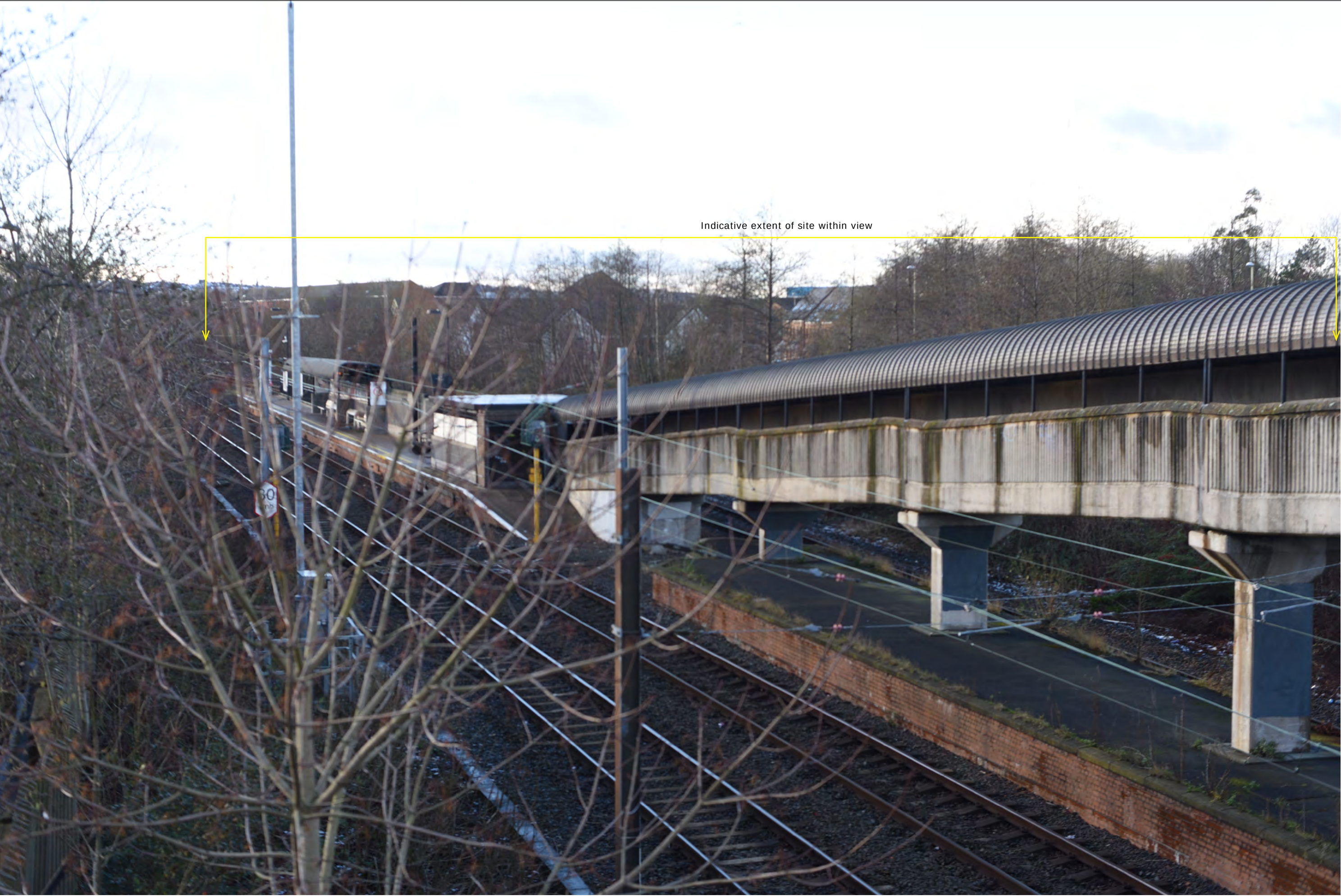
Viewpoint 3 - View west from the overbridge at Station Road
